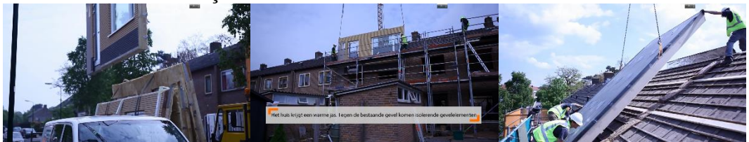
Figure 5: Installing prefabricated roof and façade elements (Sav, 2014).
