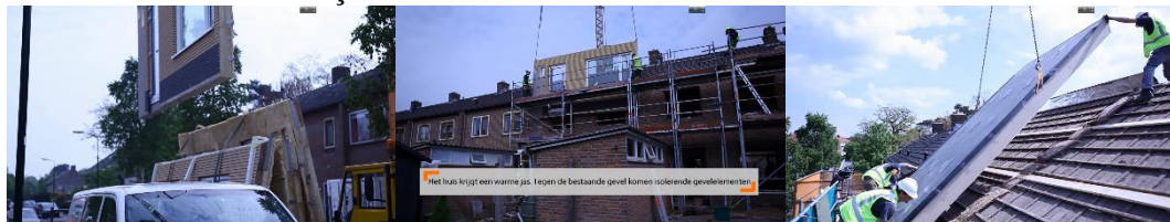
Figure 5: Installing prefabricated roof and façade elements (Sav, 2014).
