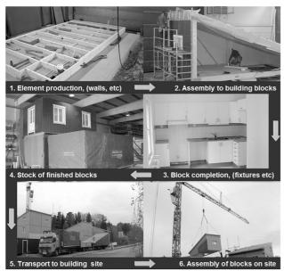
Figure 1: Volume element prefabrication and assembly.
