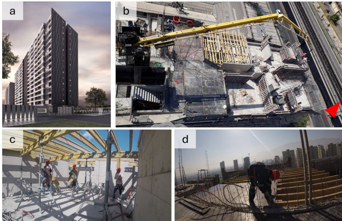
Figure 2: Case Study. (a) Building North Façade (render); (b) Plant view during reinforced concrete rough works; (c) Workers installing slab formwork beams; (d) Workers installing slab formwork panels.
