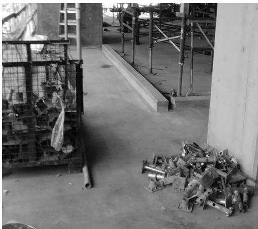
Figure 3: Waste belonging to Webcor Concrete that required removal
