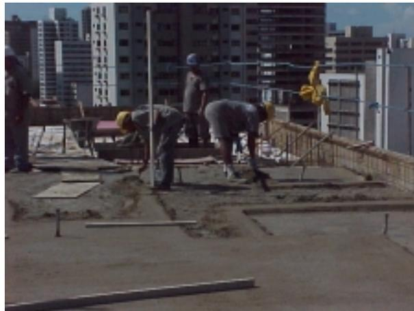
*Figure 3: Floor screeding and setbacks for brick walls positioning*
