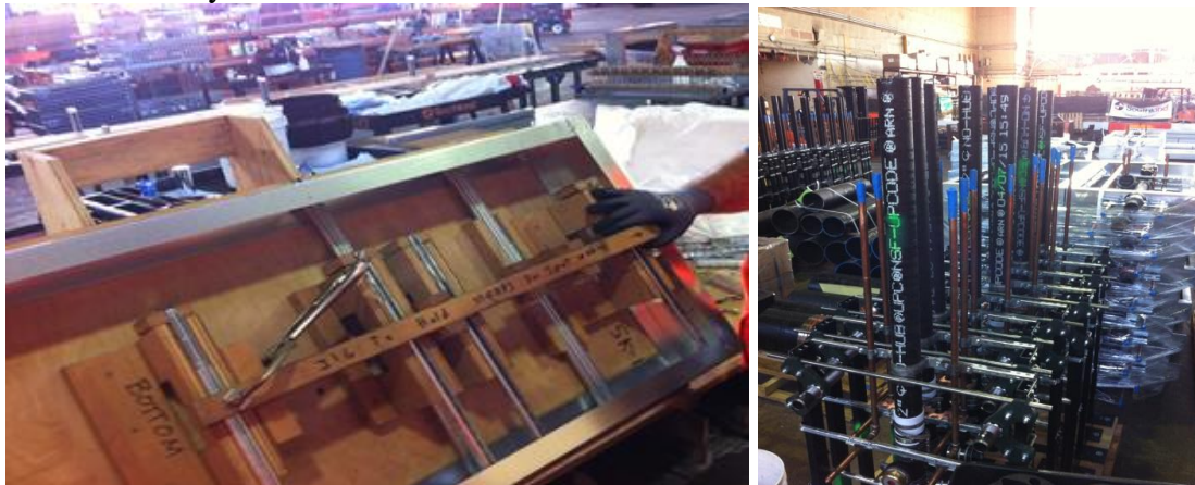
Figure 2 Welding jig on the left and stock of prefabricated modules on the right
