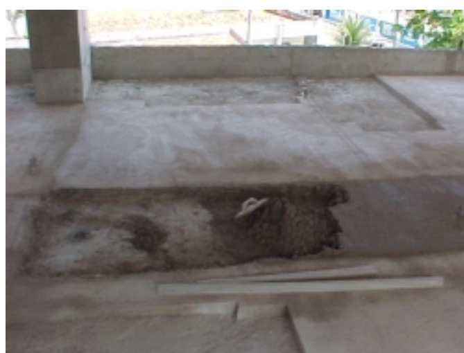
Figure 2: Floor screed executed with 50mm thickness
