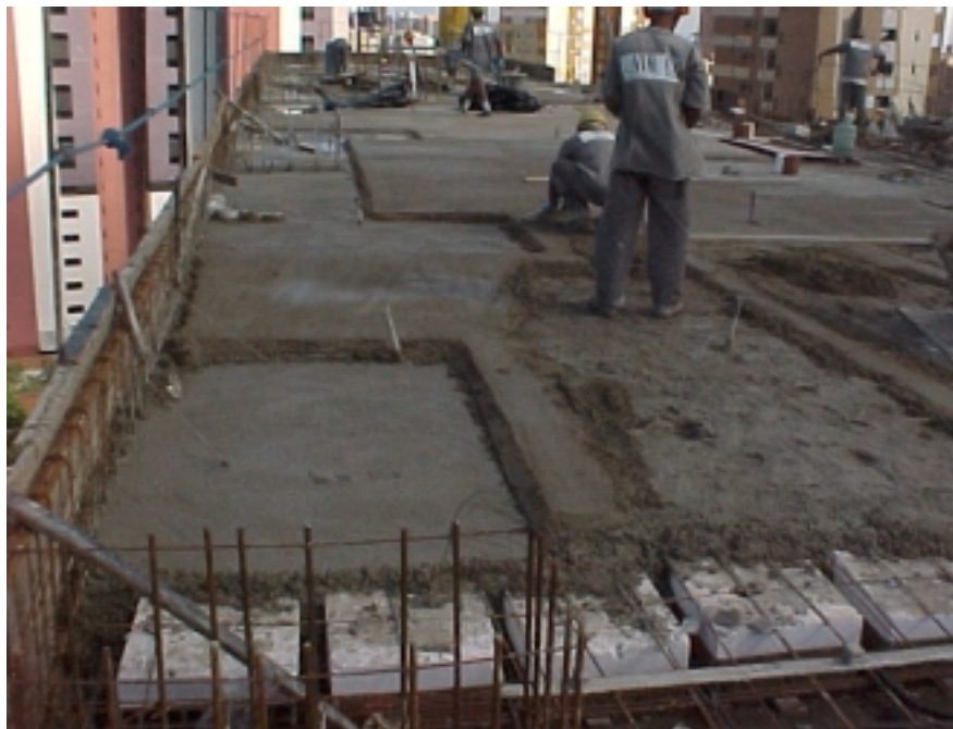
Figure 4: Molding of slab with concrete mixed on site
