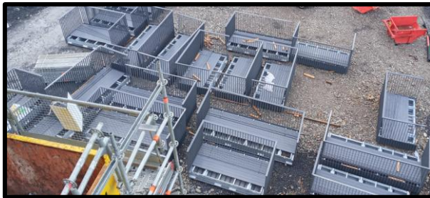
Figure 1: Balconies awaiting installation
