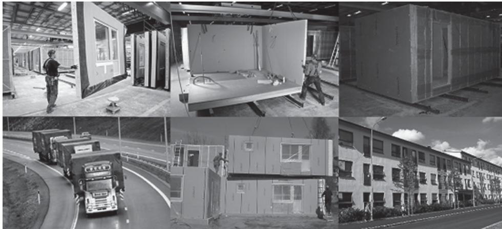
Figure 2: Manufacturing and assembly of volume elements to a finished house in TVE prefabrication
