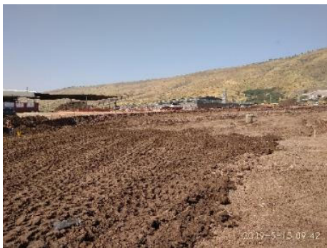
Figure 4: Location waiting for spreading operation
