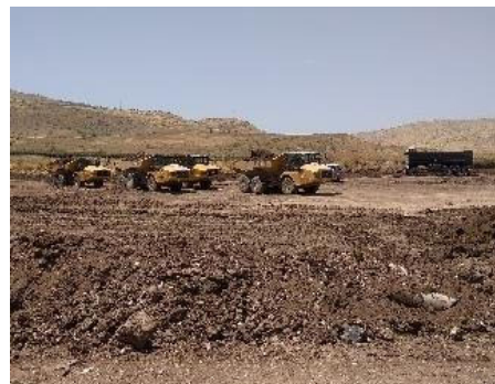
Figure 5: Trucks with material supply waiting
