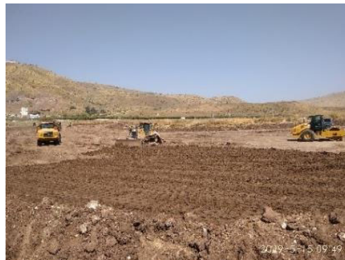
Figure 6: Compactor waiting for spread operation to finish
