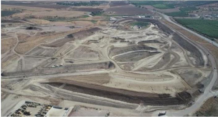
Figure 2: Picture of water reservoir under construction
