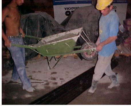
Figure 3: Stock of tracks interrupting the work flow at the site
