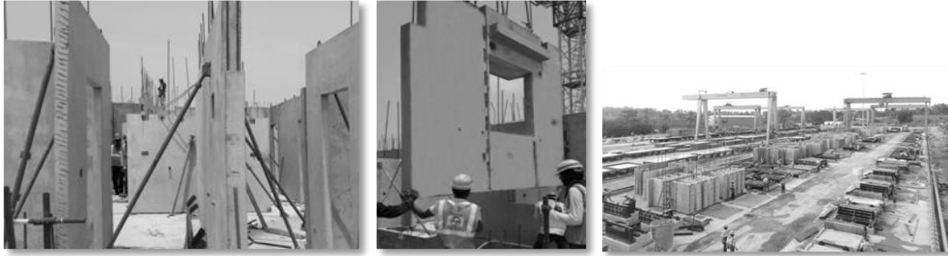
Figure 16: Precast Erection Figure 17: Precast Yard
