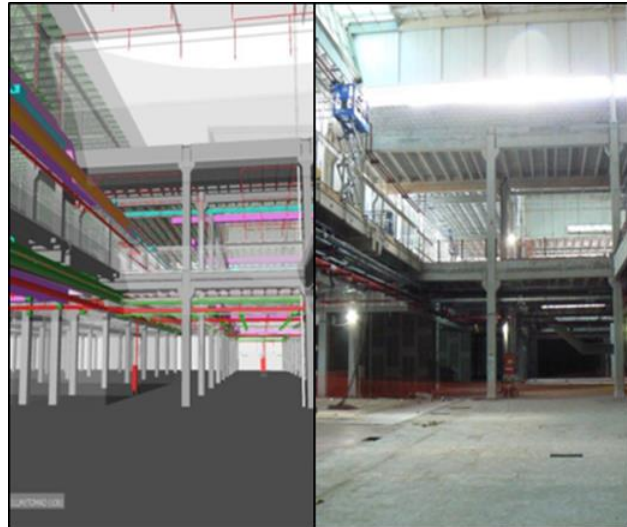
Figure 6: BIM coordination model x Site picture (Case Study I)
