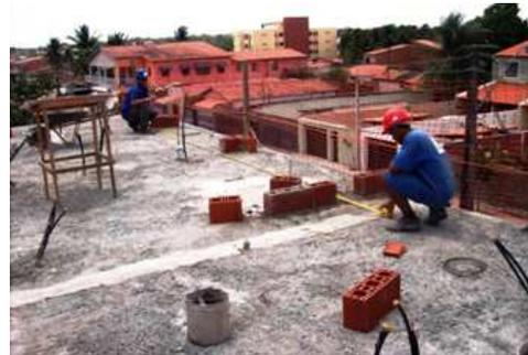
Figure 11: Marking the masonry
