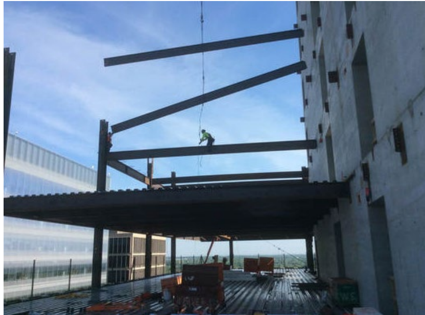
Figure 1: Christmas-treeing Method During Steel Erection (Source: Steel Erectors Association of America, 2018)
