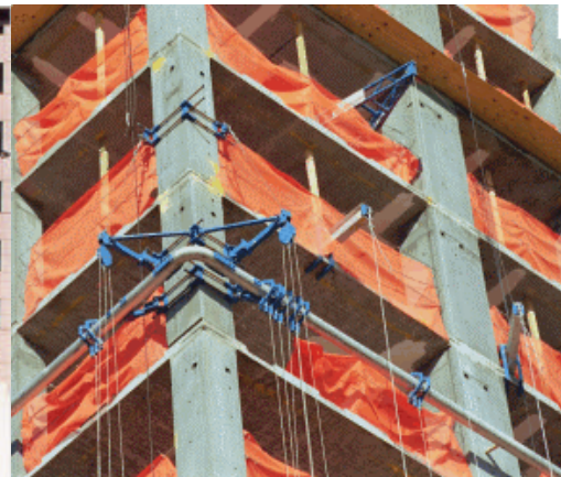
Figure 8: Corner Detail of Monorail
