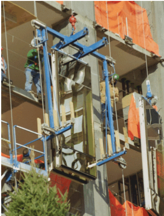
Figure 9: Hoisting Car
