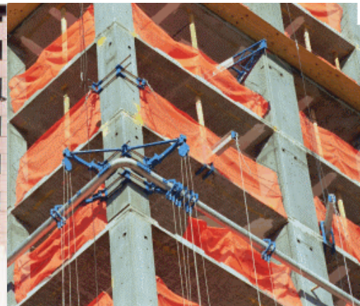
Figure 8: Corner Detail of Monorail
