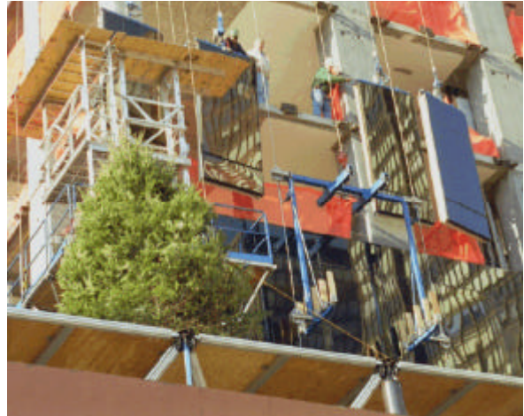
Figure 6: Hoisting Carriage and Cable-guide System
