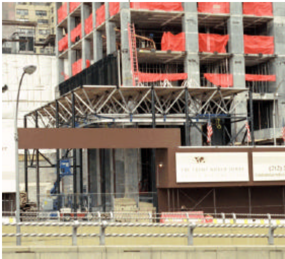
Figure 3: Aluminum Space Frame
