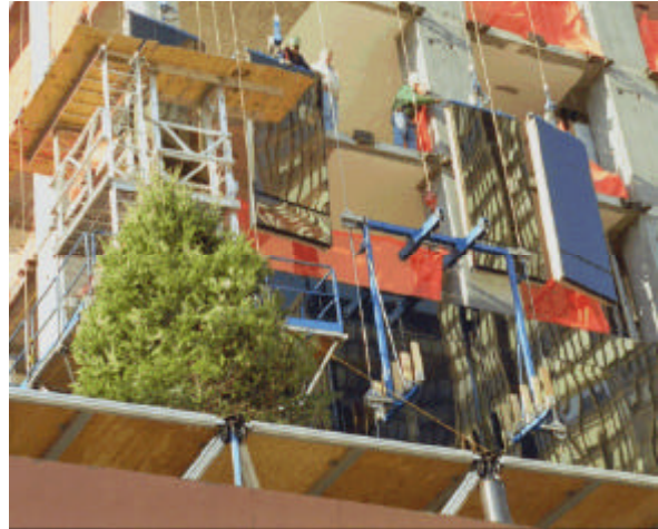
Figure 6: Hoisting Carriage and Cable-guide System
