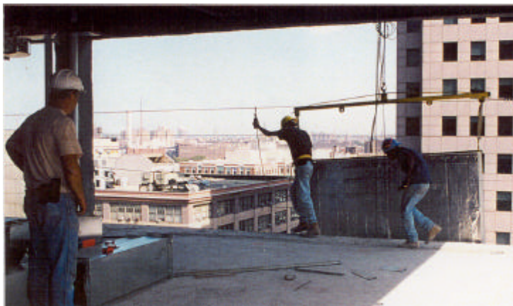
Figure 7: Walking a Panel (picture from other site)
