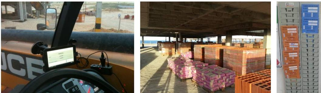
Figure 7: Tablet in a telescopic forklift, jobsite supplied and material *kanban*
