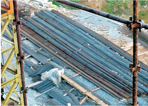
Figure 4: Piles of straight rebar
