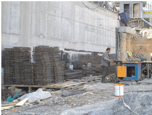
Figure 5: Piles of cut & bent rebar
