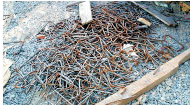
Figure 3: An example of material waste resulting from cutting uneconomical shapes
