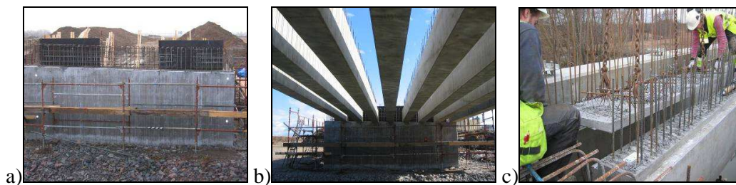
Figure 2: a) Substructure. b) Prefabricated beams. c) Prefabricated slabs
