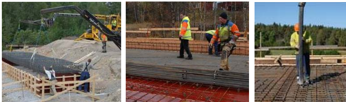
Figure 4: (a) Reinforcement cage, (b) Rebar carpet and (c) SCC
