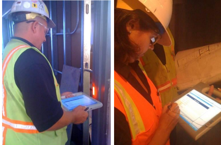
Figure 8: Barcode Scanning and SCM Status Transferring from Field to VDC Database
