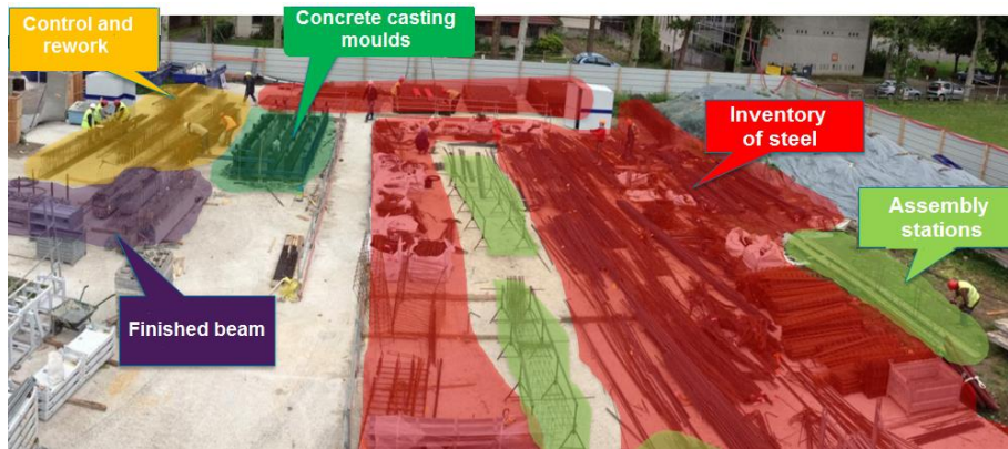
Figure 4 : Initial state of the assembly of steel beam reinforcement
