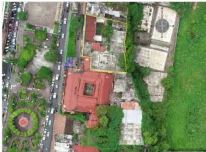
Figure 3: Topographic survey of the cathedral.
