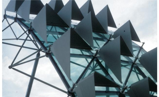
Figure 7: Mock up of aluminium sunshades and their fixing to the glazing system.
