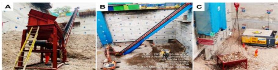
Figure 6. Operation of the conveyor belt and bucket crane.
