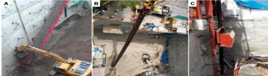
Figure 4: Alternatives to remove material for the seven, eight and nine basements.
