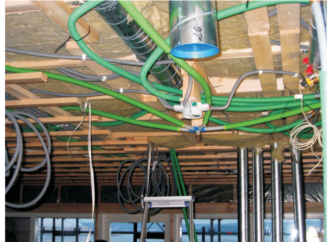
Figure 9: Complementary site work on installations in sub-ceiling.
