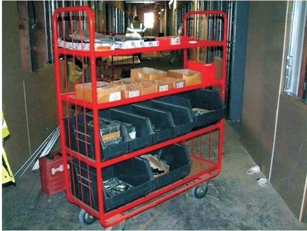
Figure 7: Mobile component trolley, with simple manual replenishment.
