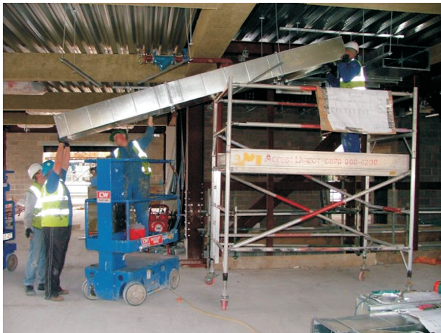
Figure 3: Conventional scaffolding and manual handling.
