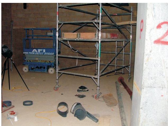
Figure 5: Unplanned workplace, conventional scaffold.
