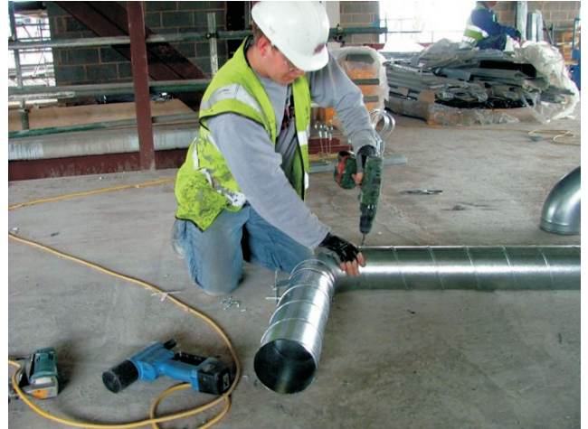
Figure 2: Working on the floor.
