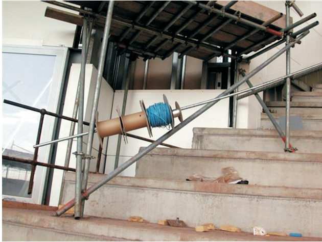
Figure 1: Improvised cable dispensing.
