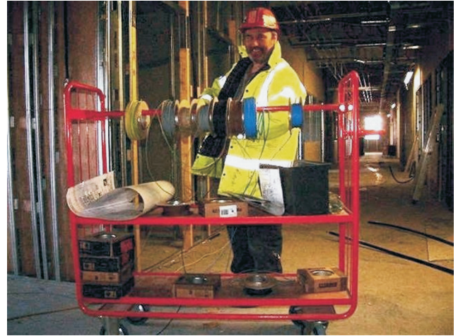
Figure 8: Mobile cable dispensing and component trolley with simple manual replenishment.
