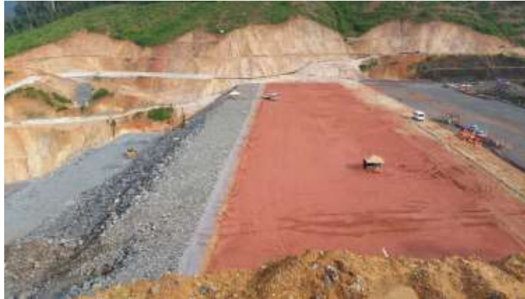
Figure 2: Dam Construction Site
