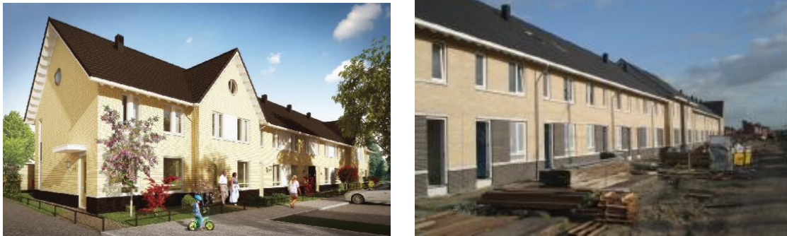
Figure 1: artist's impression and construction site
