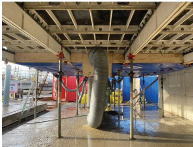
Figure 7: Slab, with hot air underneath
