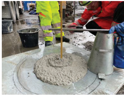
Figure 1: Controlling the workability of the fresh concrete
