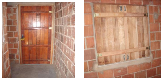
Figure 1: (a) Batten door used in PS1; (b) Window used in PS1
