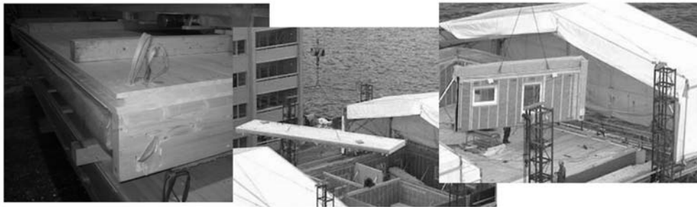
Figure 1: Prefabricated timber floor and wall elements used for multi-storey housing
