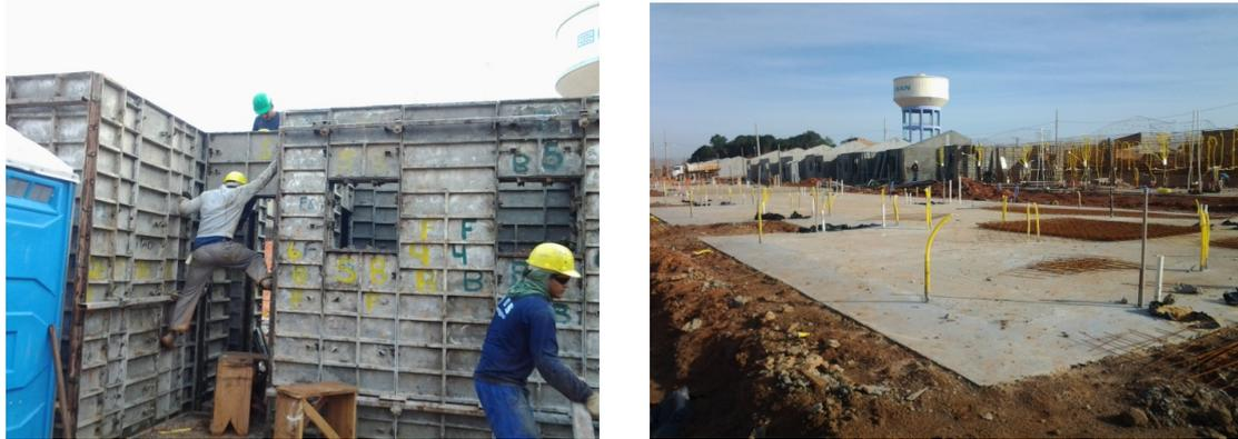
Figure 7: – Examples of improvisation: worker supporting himself on the concrete wall formwork (left) and inadequate electricity pipes in the raft foundations (right)
