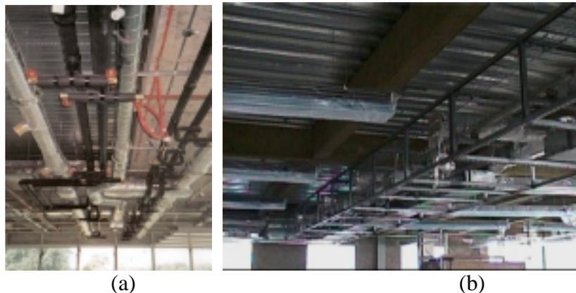
Figure 1: (a) Traditional horizontal distribution of building services (b) Installed prefabricated horizontal distribution units
