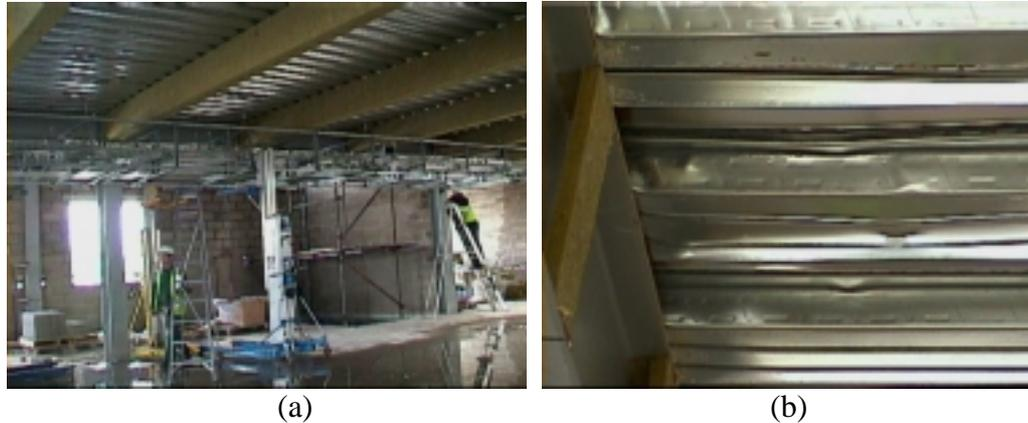
*Figure 5: (a) Units being installed on site (b) damaged floor-pans causing installation problems*
