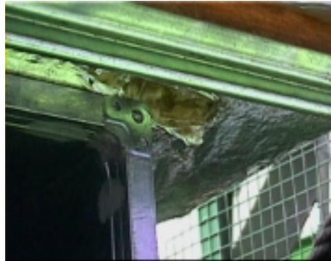
*Figure 6: Damaged insulation within horizontal services distribution module*
