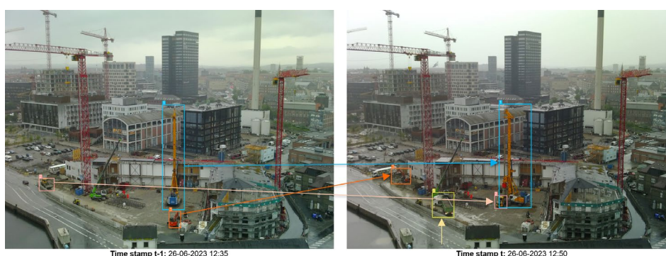
Figure 7. Detection and tracking of machines between two consecutive images
