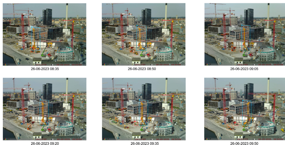
Figure 6. Detection of equipment and its operation status on 26-06-2023
