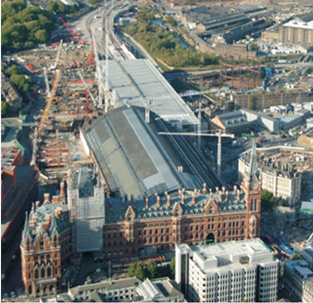
Figure 1: Channel Tunnel Rail Link Contract 105 at St. Pancras Station
