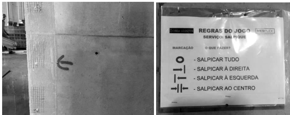
Figure 1: Example of spray marking of the kind of rough cast and its explanatory sheet
