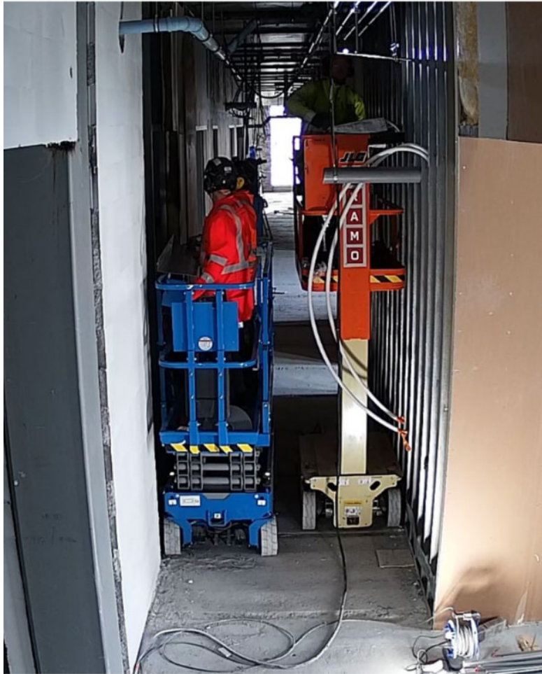
Figure 2: Two crews working side-by-side in the same takt area
