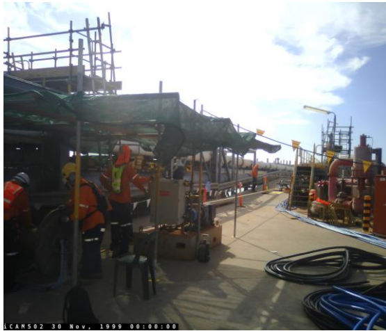
Figure 5. Use of winch
