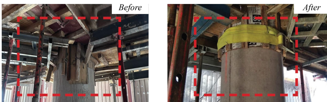
Figure 3: Improvement of falsework and formwork for column
