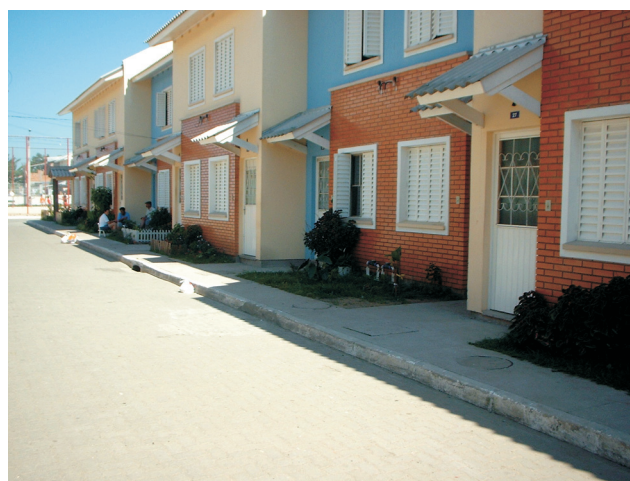
Figure 4: New dwellings, part of PIEC
