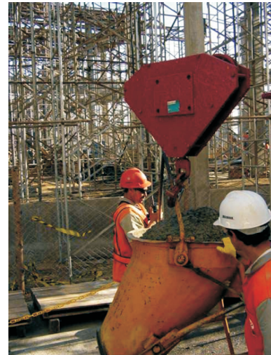
Figure 2: The pulley of a crane involved in accident 2.
