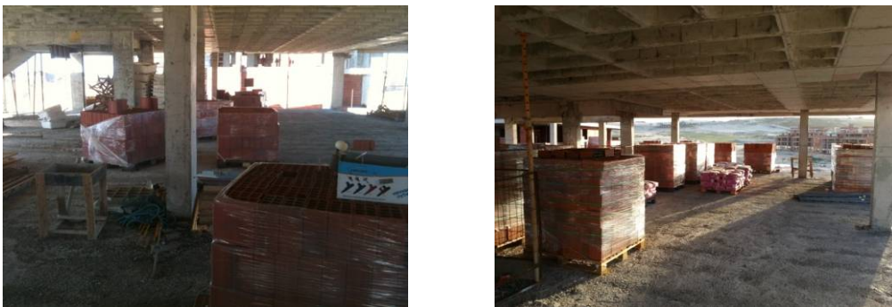
Figure 9: Jobsite before and after the implementation of the heijunka system.
