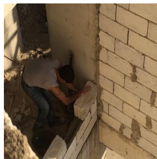
Figure 7: Working in awkward and restricted space
