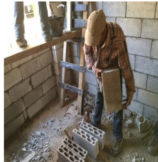
Figure 4: Worker exposing his back to potential injuries
