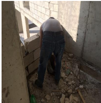
Figure 3: Involvement of a worker lifting a heavy object
