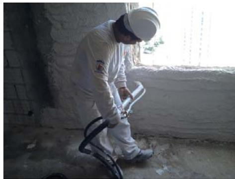
Picture 5 (b): Plasterer projecting gypsum in the wall.
