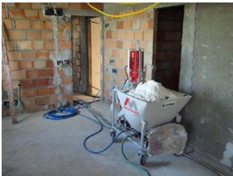
Picture 5 (a): Gypsum machine projector.
