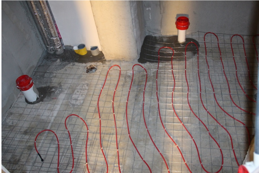
Figure 4: Typical bathroom, post-demolition, with tubing laid for in-floor heating
