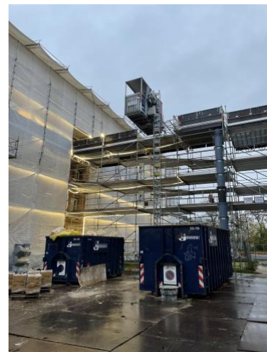
Figure 2: Façade scaffolding and scaffolding between Buildings B1 and C1.
