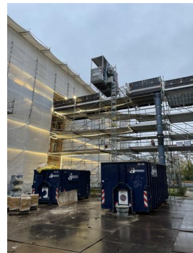
Figure 2: Façade scaffolding and scaffolding between Buildings B1 and C1.
