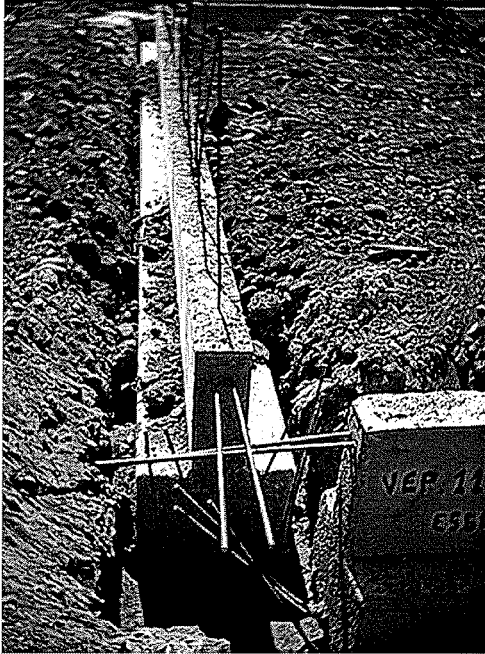
Figure 1. Prefabricated Foundations
