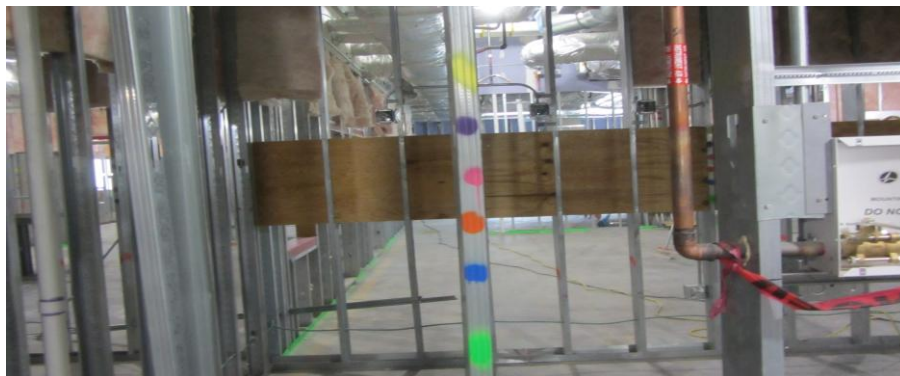
Figure 8: Color-coded visual management system on metal studs indicating completion status of different trade work (Akron Children's hospital). Photo by Z. K. Rybkowski.
