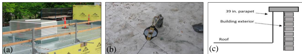
Figure 1: Suggested fall-protection systems (Rajendran and Gambatese, 2013)
